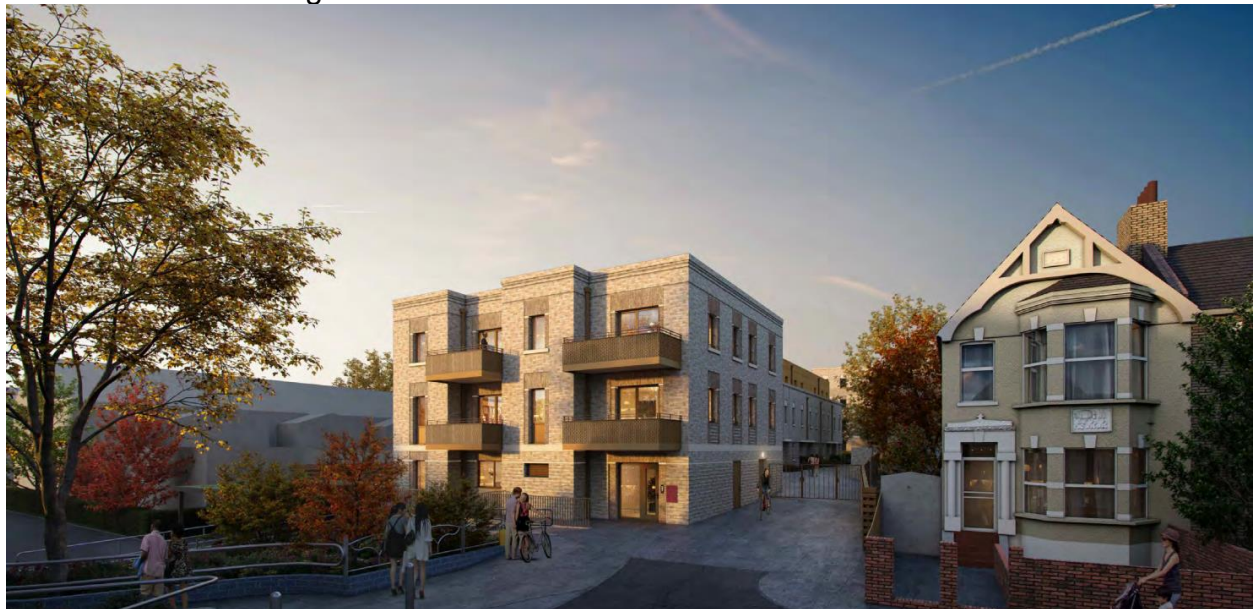
Street view of Building D1 and Brunel Walk seen from Kirkton Road
