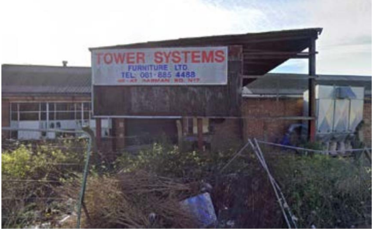
View from roundabout on north-west corner
