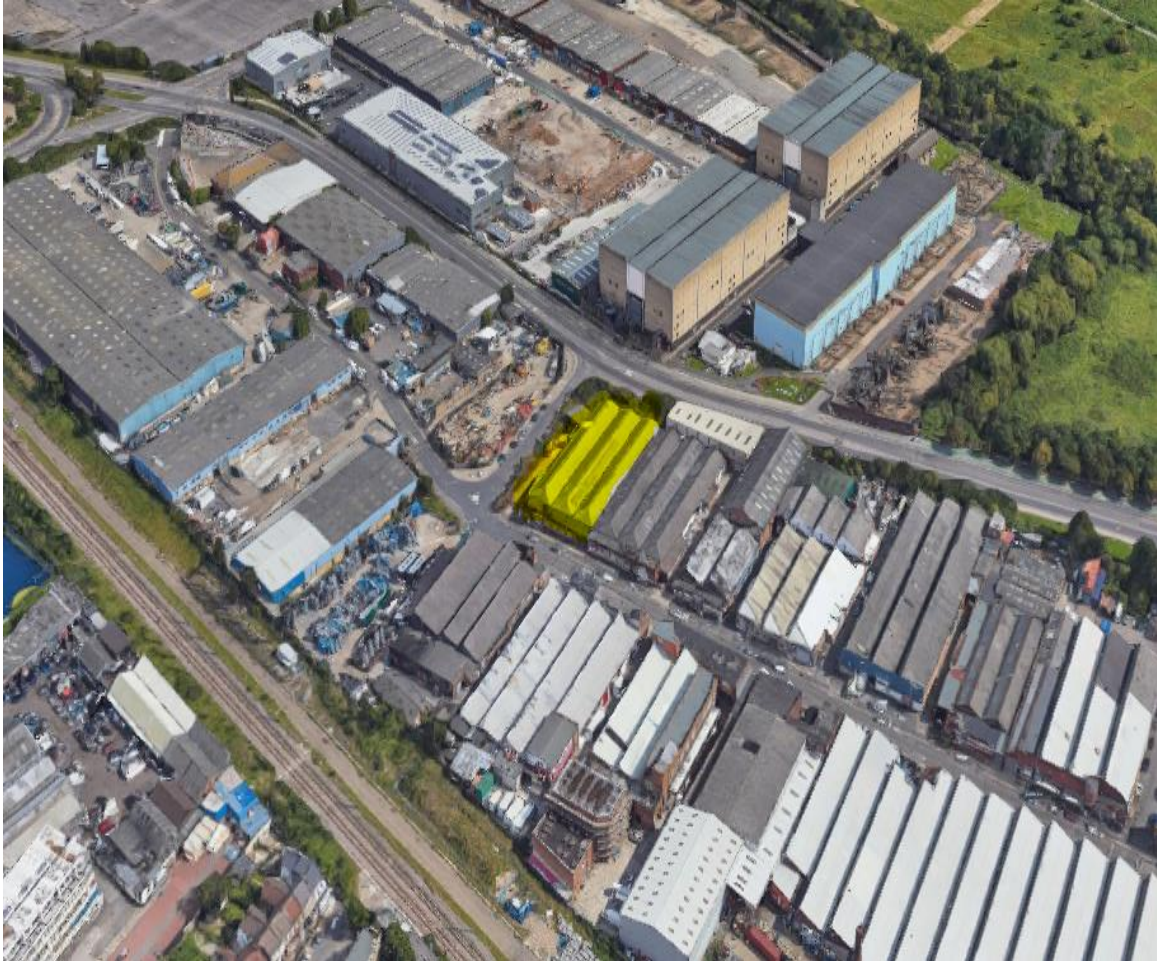
Image 2 Aerial view of the site
